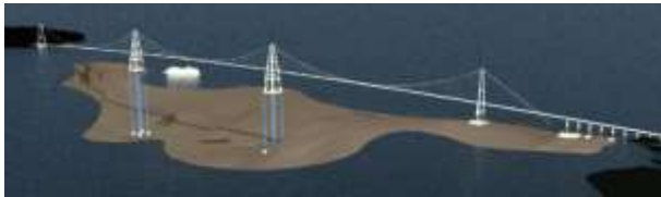
Figure 2. 3D view of bridge depicting concept for floating foundations midfjord. Courtesy NPRA
