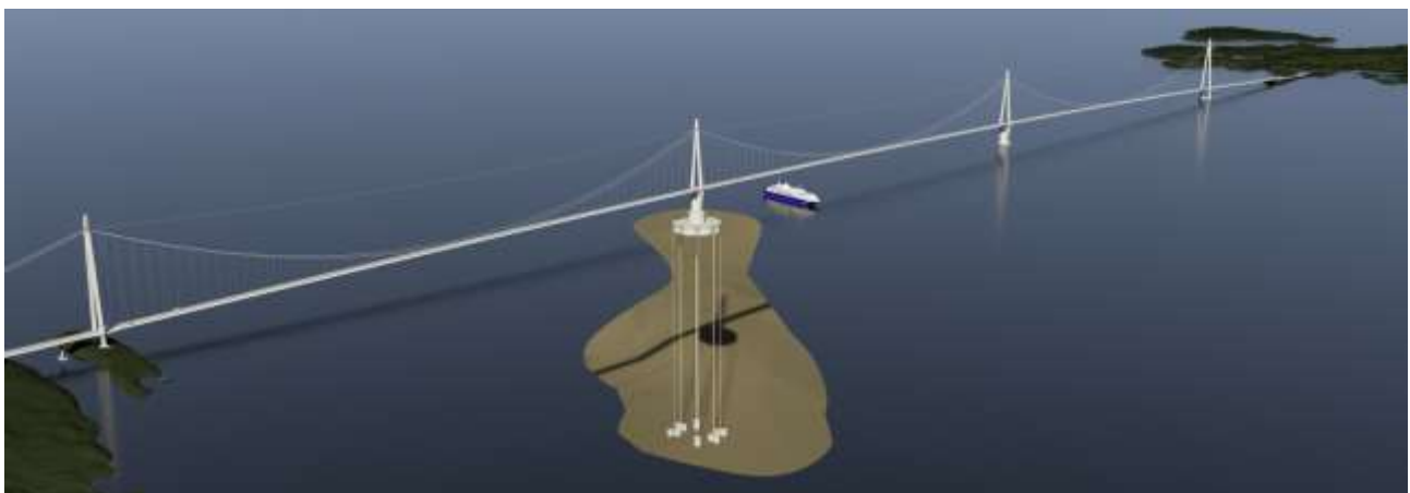
Figure 1. Rendering example of the multi-span suspension bridge on floating foundations crossing the Bjørnafjord.
