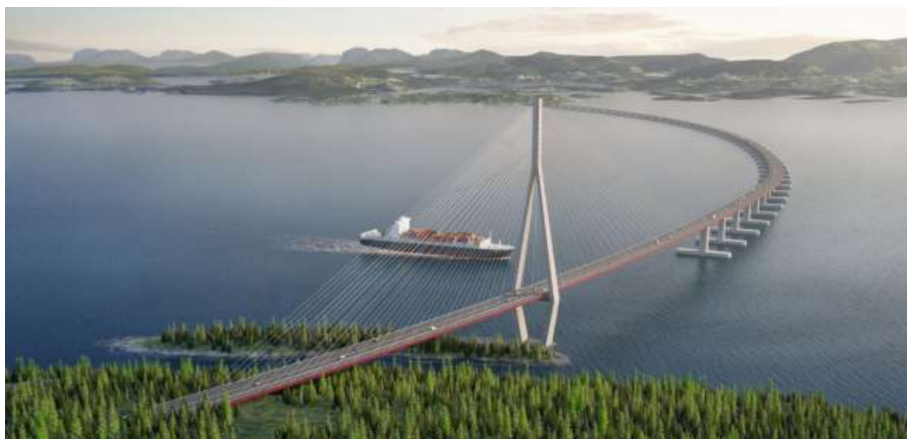
Figure 1. Bjørnafjorden floating bridge concept (Illustration. Statens Vegvesen / Vianova / Baezeni)
