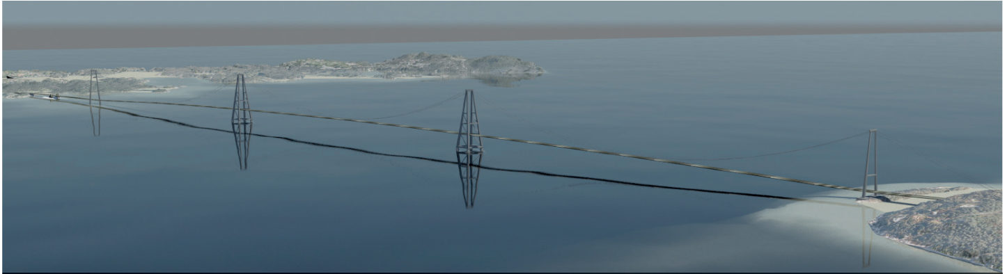
Above: The proposed bridge has two tension leg floats and two bottom-fixed traditional towers. (Courtesy NPRA). Below: The first five lateral eigenmodes of the bridge
